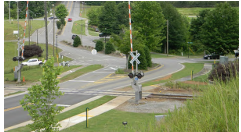
Howell Bridge Road Looking West Towards I-575 Across Georgia Northeastern Railroad
