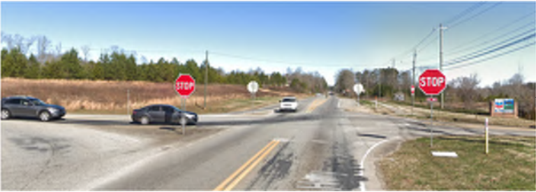
Howell Bridge Road at Ball Ground Highway
